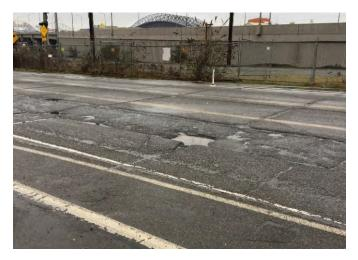
Figure 4: Deteriorated Roadway Conditions along the Project Corridor
